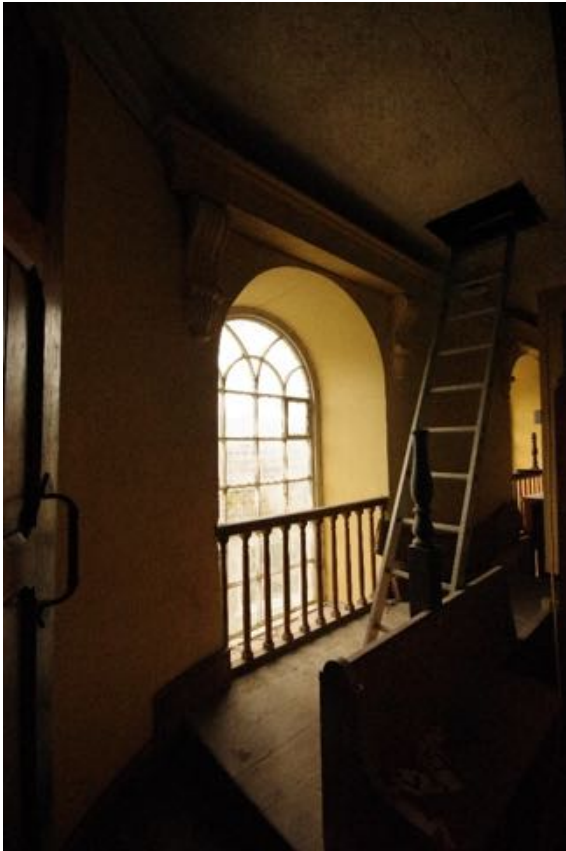
Fig 20 Space behind the organ showing original window in the apse with decorative consoles and entablature over the opening.
