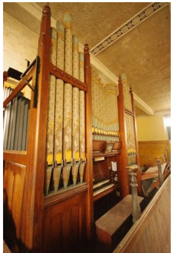
Fig 15 Organ situated above the rostrum. The organ frontage is to remain visible from the main church space.
