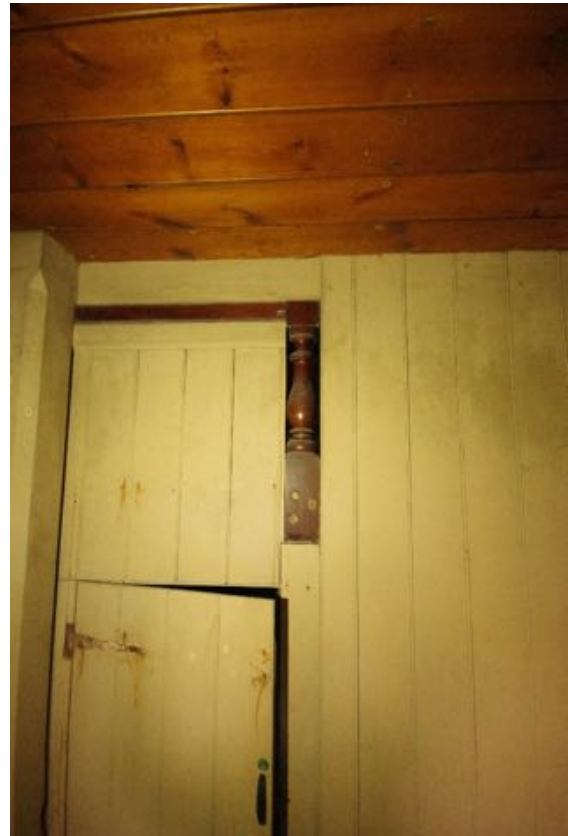
Fig 18 Remains of earlier rostrum or pulpit within the rear of the current late 19th century arrangement.
