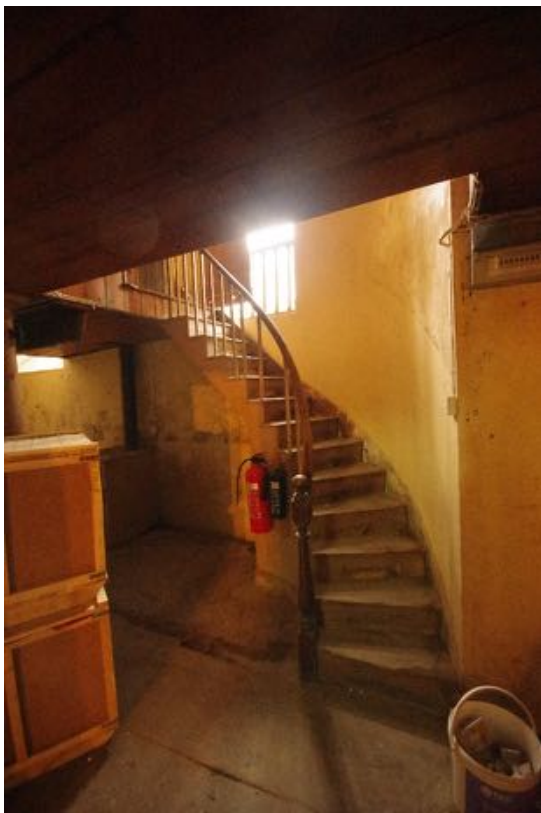
Fig 17 Curved timber staircase behind rostrum.
