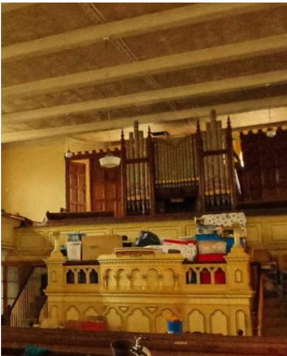
Fig 21 View of the timber panelled partition located beside the organ.
