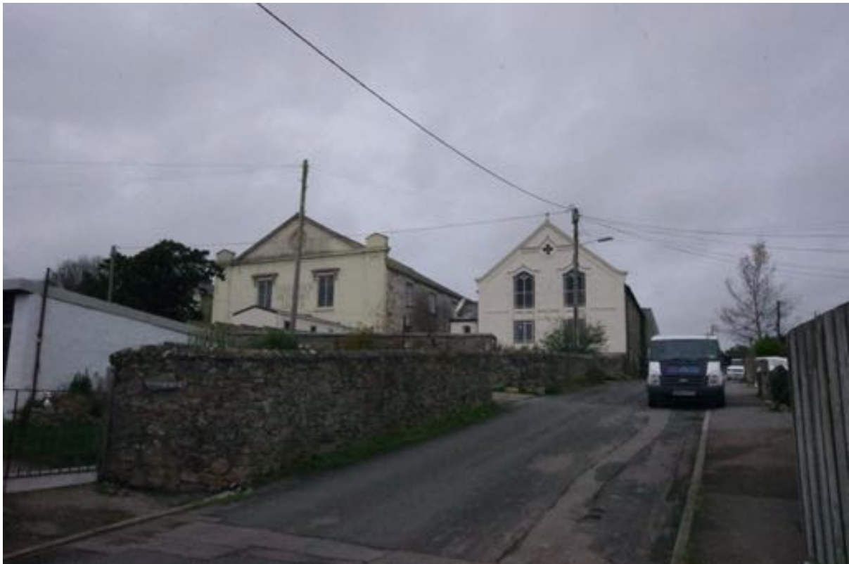
Fig 6 Carharrack Methodist Church (left) and Sunday School (right) as viewed from the road.
