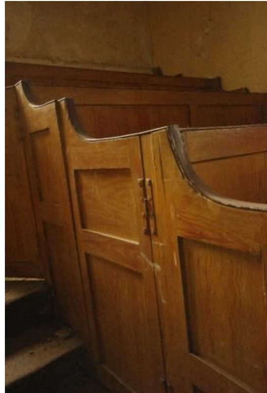
Fig 14 Box pews which are proposed to be removed and used in the restoration of the remainder of the gallery.
